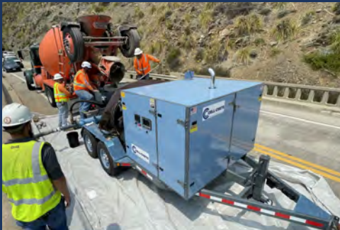
Towable Inline Pump (Wet Mix) – Enables mobility and efficient pumping.
